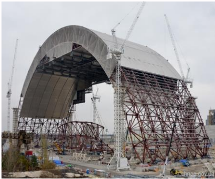
Installation of the NSC in the "safe" zone of the construction site
