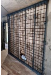
Installation of reinforcement of wall panels
