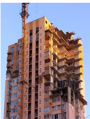
September 08, 2022 (concreting of poles and floor slabs)
