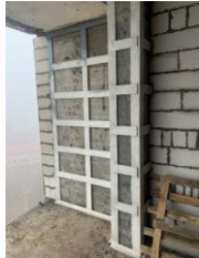
Installation of reinforcement of wall panels
